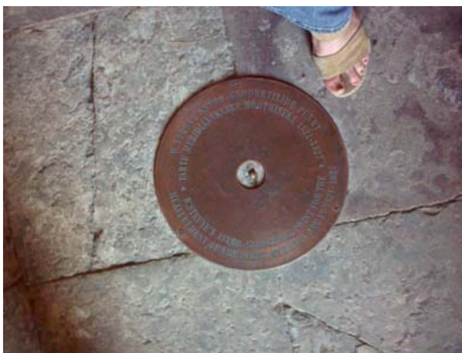
Fig. 7.1 – Mark indicating the Struve Geodetic Arc at the Astronomical Observatory, University of Tartu. The arc stretches across 10 countries from Norway to the Black Sea. It constituted the first accurate measurement of a long segment of a meridian. The survey was carried out between 1816 and 1855 by the astronomer Friedrich Georg Wilhelm von Struve (1793-1864). Struve supervised the survey from the University of Tartu, where he worked from 1813 to 1839.
